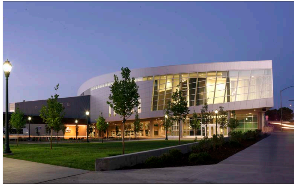
ABOVE: The newly-constructed Spokane Convention Center features 13 surveillance cameras and six, multi-channel DVRs. Photo courtesy of SPFD.
